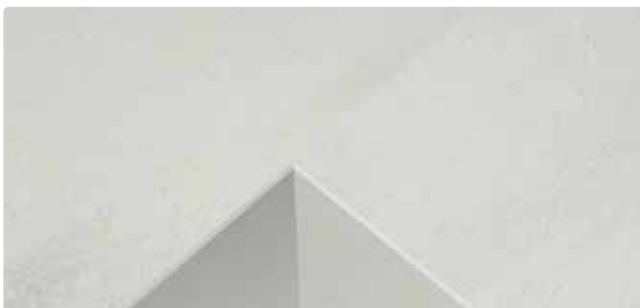
Detail seamless corner joint at Corian.* Note: despite seamless joint, decor is not continuous.
